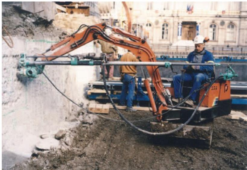
***Pneumatic Rock/Concrete Drill***
